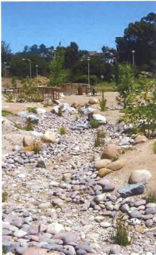
Dry Streambed Swale
